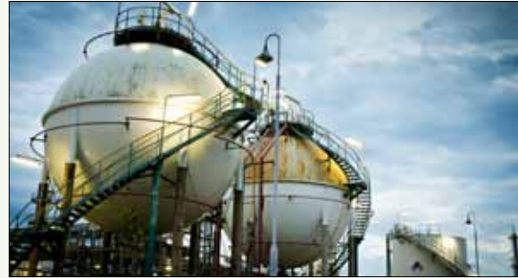
Korea Gas Corporation Substation 21 in Pyeongtaek
