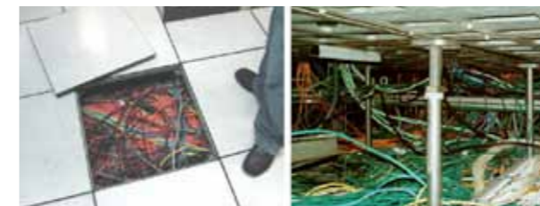
[Figure 3] Cable distribution system in Data Center
