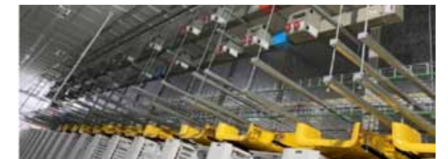
[Figure 4] Busduct distribution system 1
