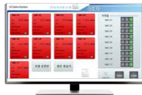
· Rack monitoring screen
